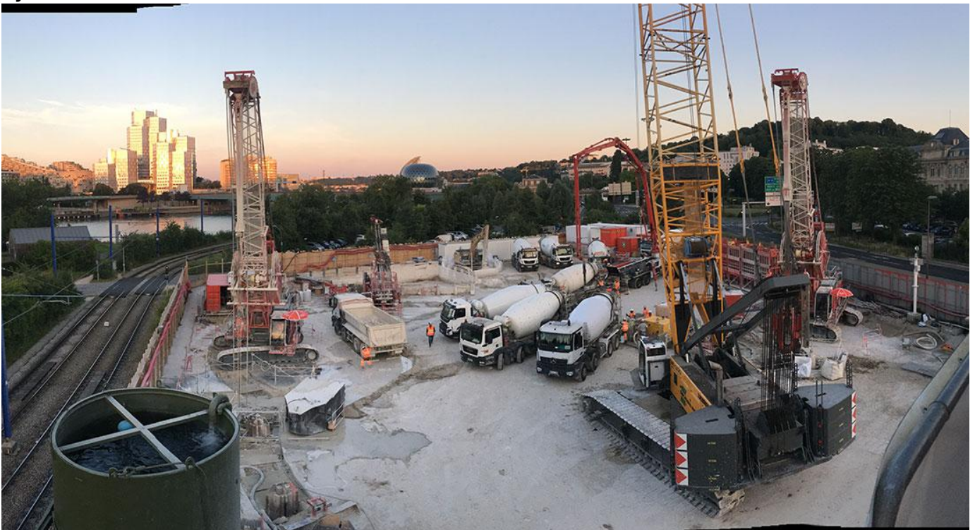
Marie DESABRES - Soletanche Bachy Vonci Construction, Sèvre, France
